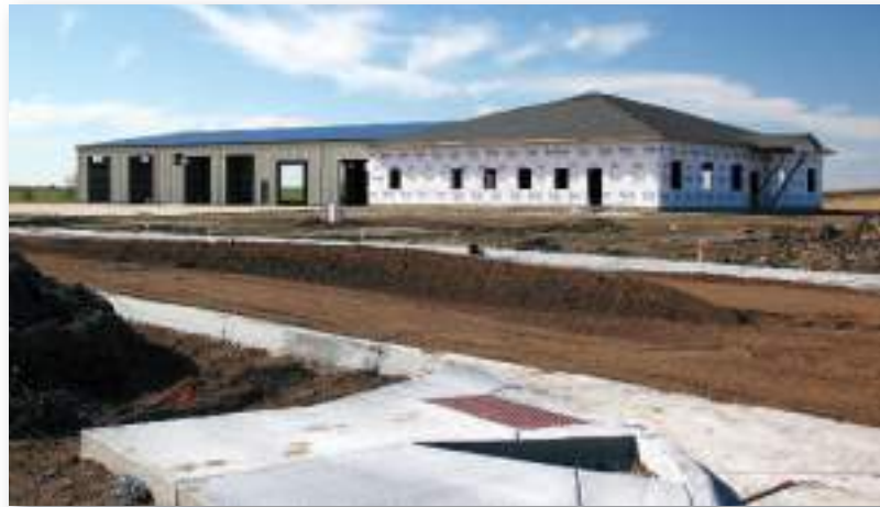
Street construction in Foundation Park and Dakota Carriers.
